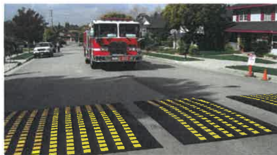
Figure 4: Temporarily Speed Tables Example
