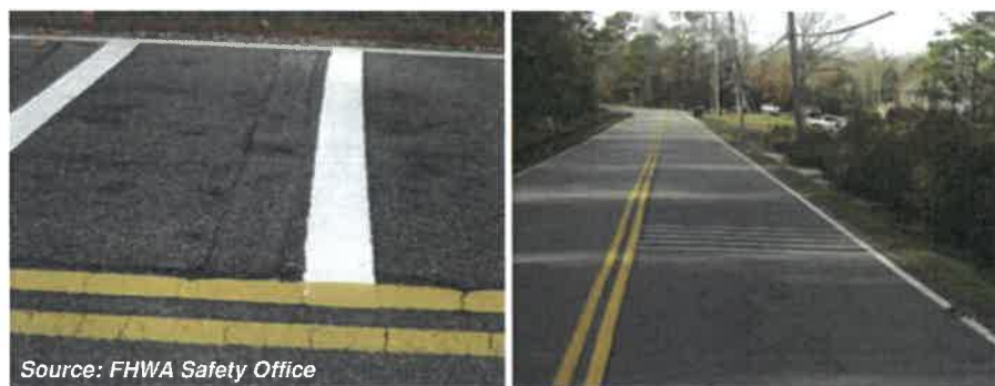
Figure 9: Traverse Rumble Strips Example
